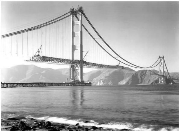
Golden Gate bridge construction - 1937
